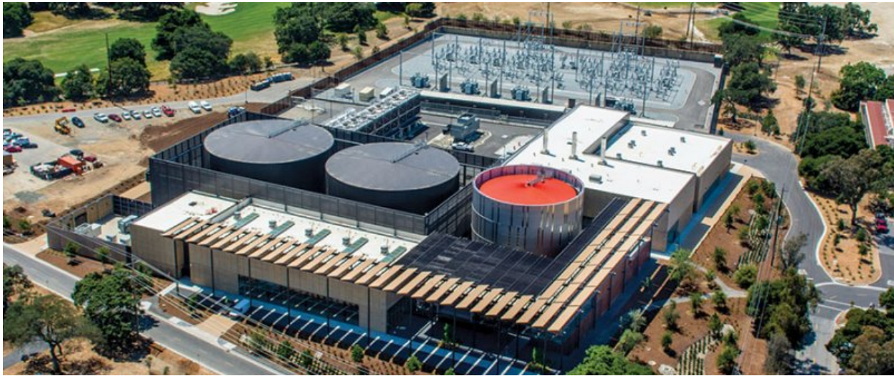
Figure 6: Aerial view of SESI
